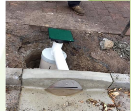
Kerb Inlet + Porous Well
